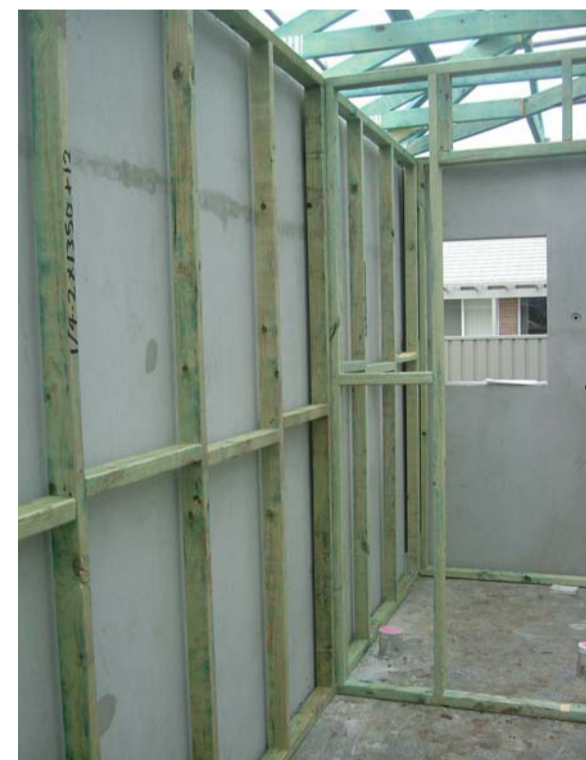
INDEPENDENT FRAMED INTERNAL WALLS, NON LOAD BEARING
