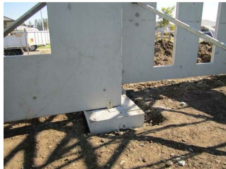
PRECAST WALL ON PRECAST PAD FOOTING
