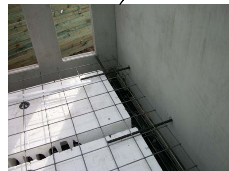
INSITU FLOOR SLAB SUPPORTS PRECAST WALL
